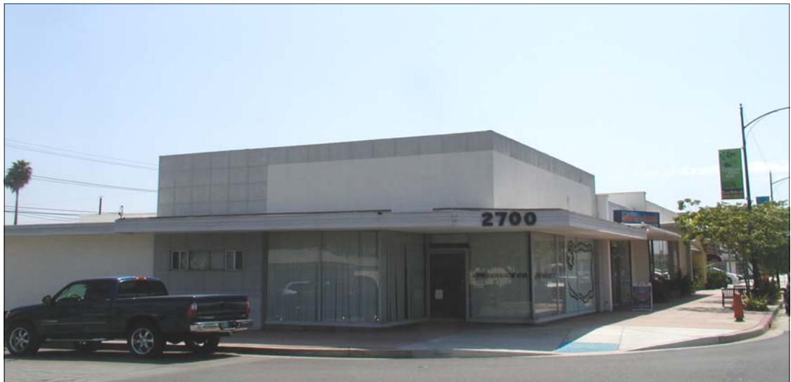
Corner Property With Signage
